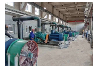
Cement Plant Project
