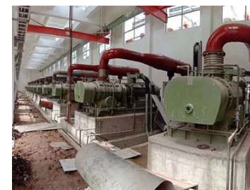
Power Plant Project
